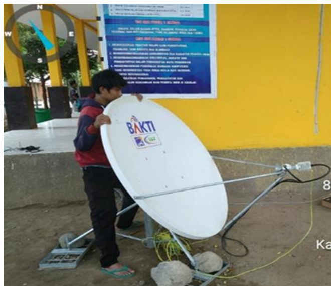
Figure 3.7. VSAT antenna pointing
