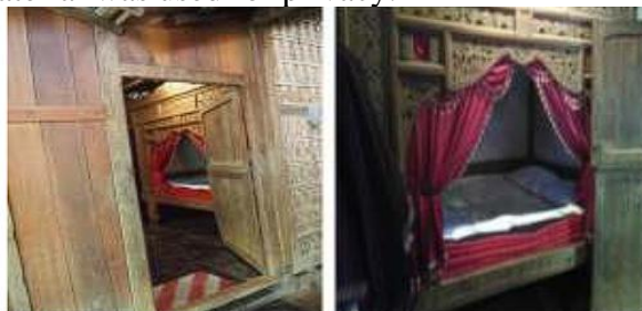
Figure 03. Mbyale in the Using Traditional House The concept of proportion is also seen in the use of building materials and decorative elements. The woven bamboo (gedheg) used as side walls, back walls and house partitions has a certain pattern that reflects visual and aesthetic balance. The interviewee stated that in rooms other than the bedroom (jerumah), single bamboo woven material was used to allow good air circulation, while in the jerumah double bamboo woven material was used for privacy.
