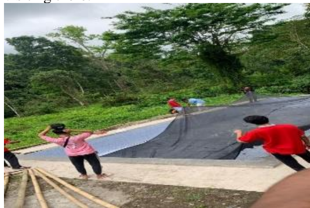
Figure 1. Installation of Paranet in the Sumberan Camping Ground Pool Area
