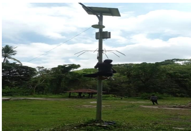
Figure 4. Installation of lighting in the Sumberan camping ground area
