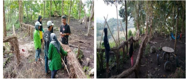
Figure 9. Making a stair handrail
