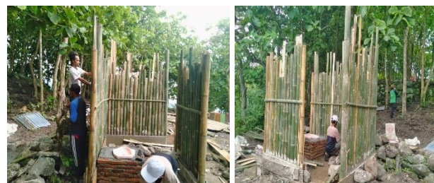
Figure 2. Construction of MCK
