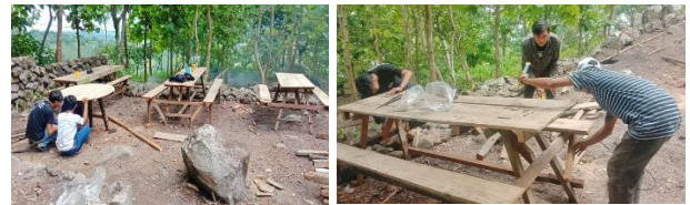
Figure 10. Construction of visitor seating
