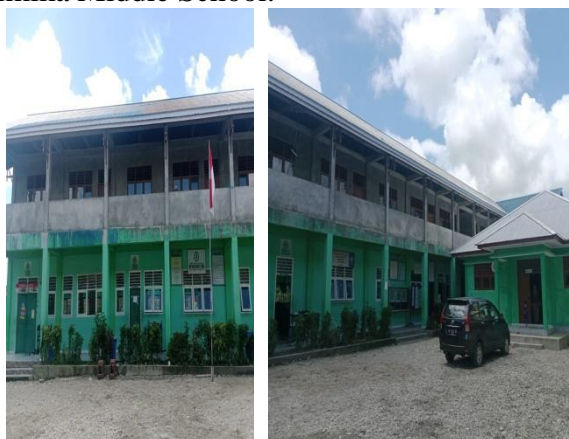
Figure 1. Condition of Yapis Branch 2 Timika Middle School
