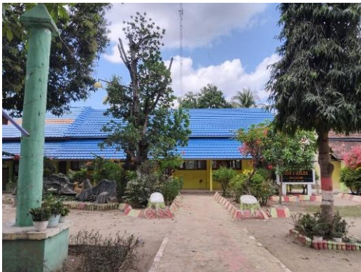
Figure 2. Condition of SDN 1 Kaleo
